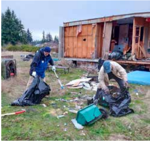
Clean-up of new Mason Street site.
