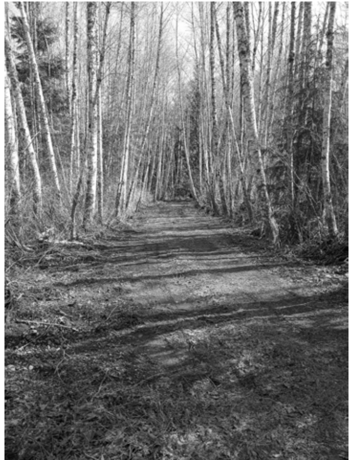
Timberton Traditional to McCormick Loop Trail widened and cleared.
